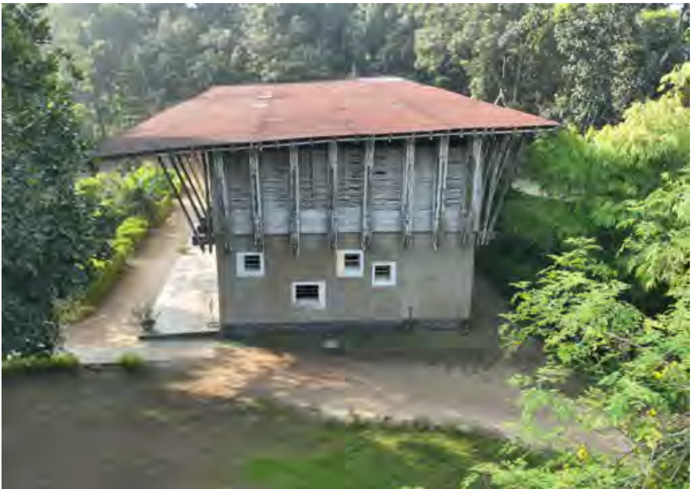
Top: Drone view of METI Handmade School, Rudrapur, Dinajpur Bottom: Western Side of METI Handmade School, Rudrapur, Dinajpur
