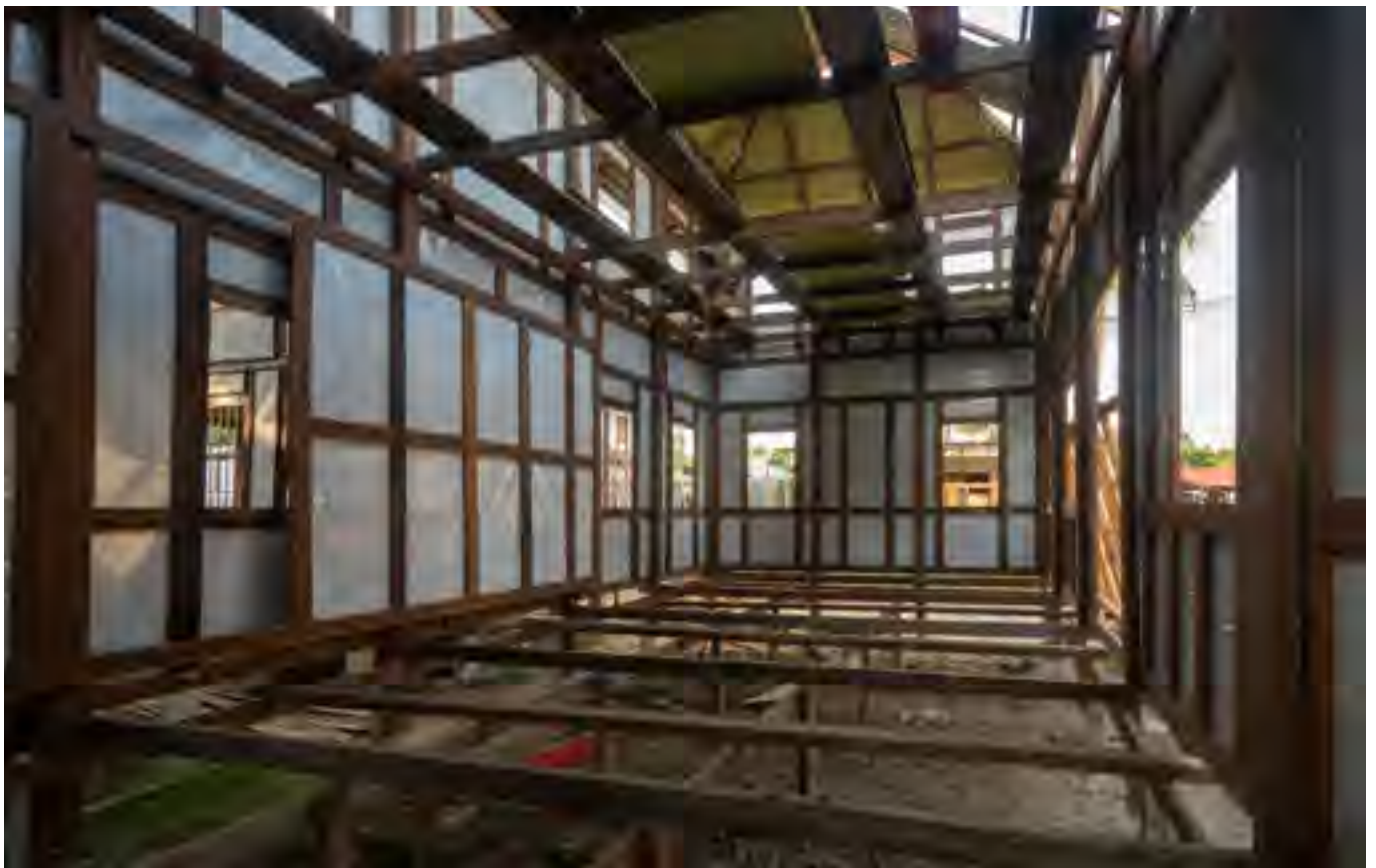
Top and Bottom: Interior Space of Munshiganj Prefabricated House, Munshiganj
