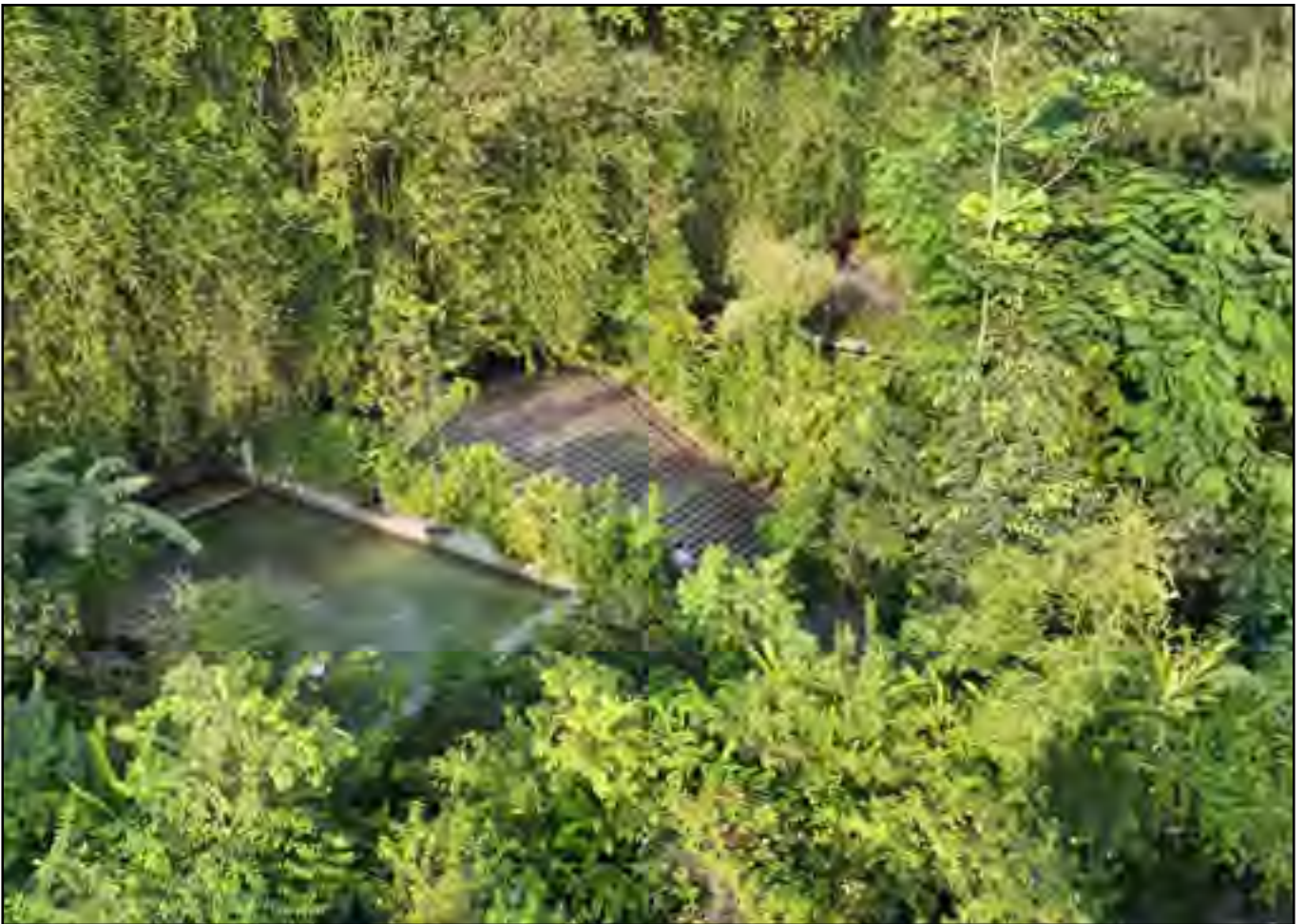
Roof Garden of Karupannya Green Field Factory, Rangpur
